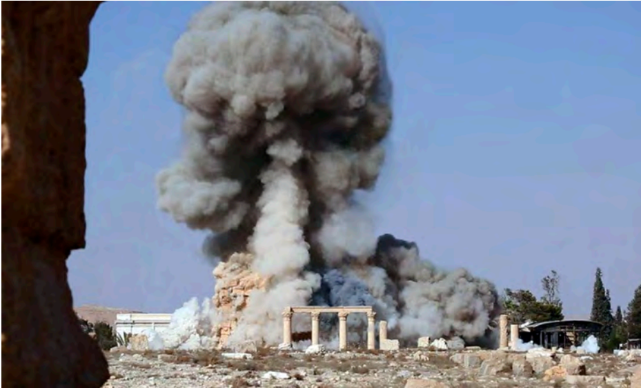
Figure 3.4 Demolition of the Temple of Bel in Palmyra by ISIS in 2015. Image: akg-images / Pictures from History
