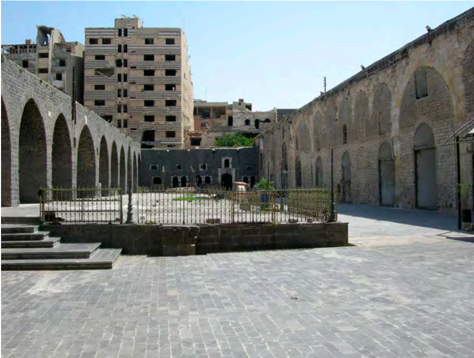
Figure 11.6a The main courtyard of the Al-Nuri Mosque. The structure is built of black basalt, the local building material of Homs. Image: Marwa al-Sabouni
