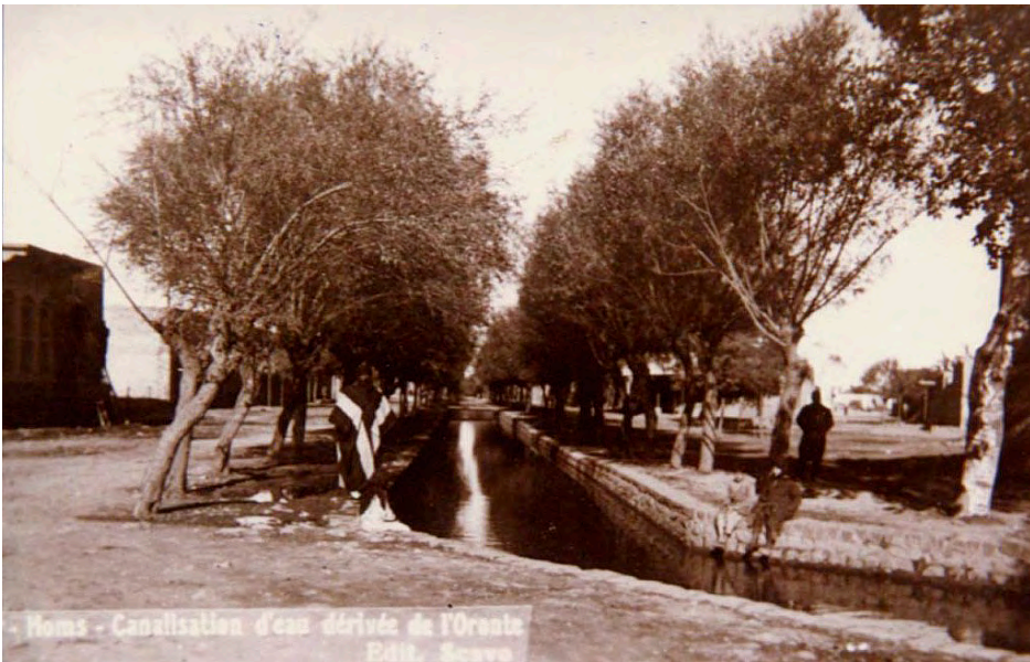
Figure 11.9b An historic photo of the irrigation canal of al-Mujahediya, a beloved part of the picturesque cityscape that was largely covered by roadways as part of so-called modern planning. Image: Courtesy of Homsstory.com
