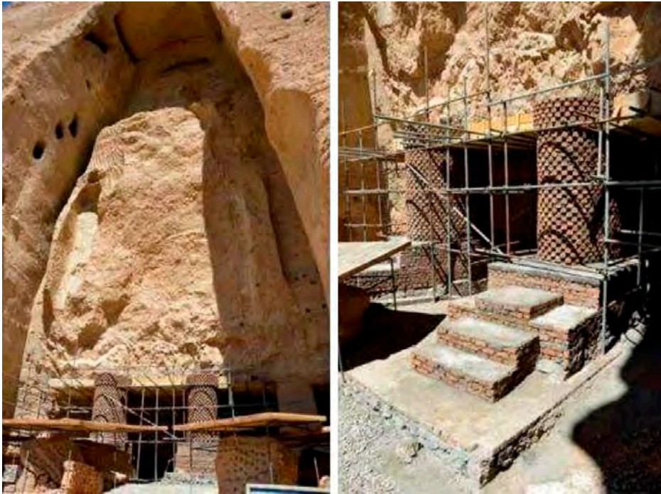
Figure 8.3 Supporting pillars for the eastern Buddha, left, with detail at right
